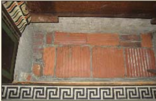
The second panel in the southeast corner was removed to reveal terracotta infill.
