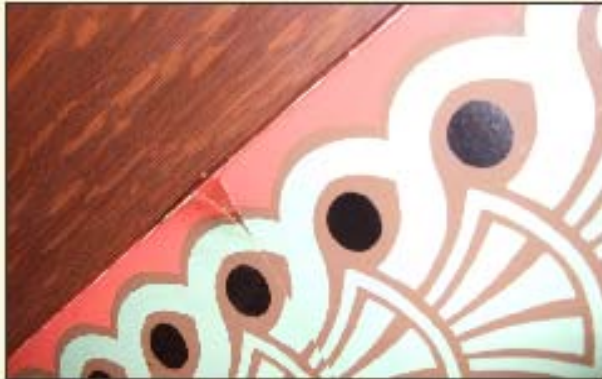
The decorative pattern on the bottom of the wood beams was confirmed to be an applied paper.
